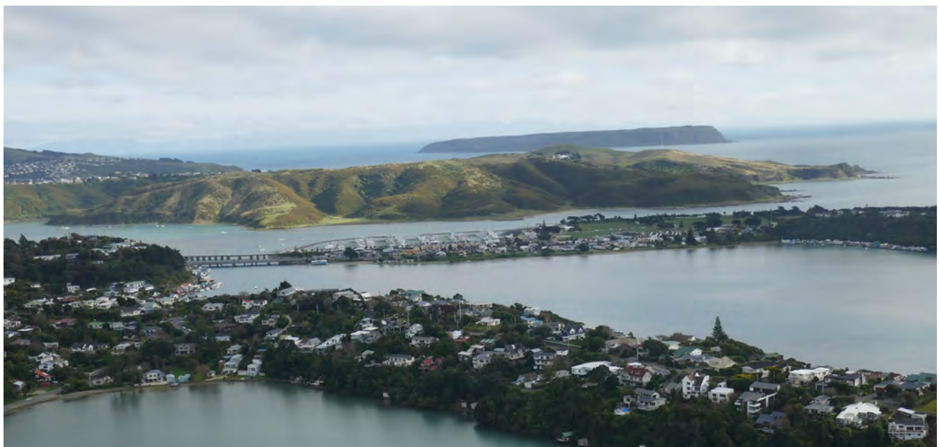
Whitireia ONFL: Coastal escarpment, seen from the west (aerial view).
